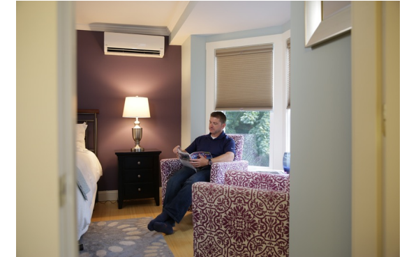
Mini-split Heat Pumps
