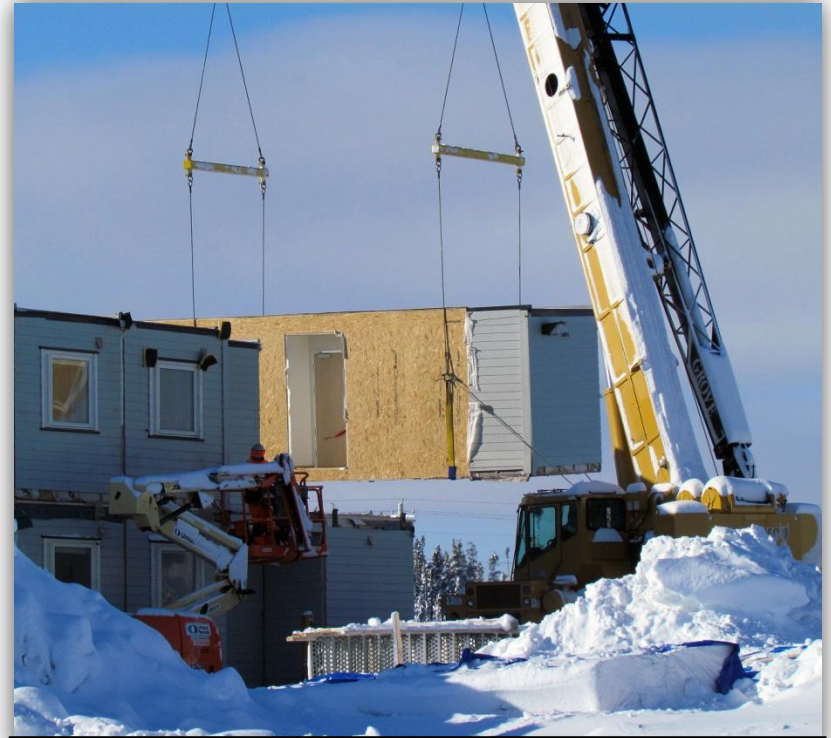
Accommodation facility construction at Granite Canal, December 2014
