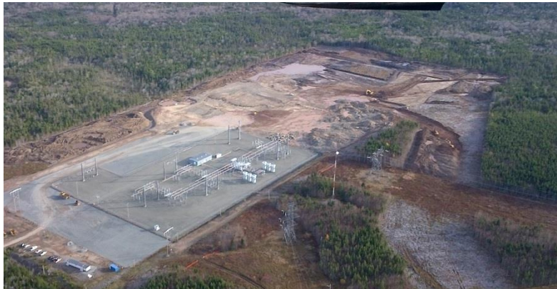
Woodbine Converter Station site (NS)
