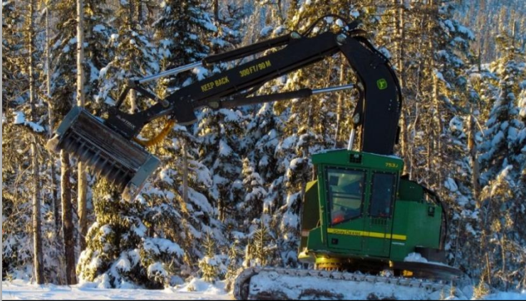
Mulcher clearing ROW in NL
