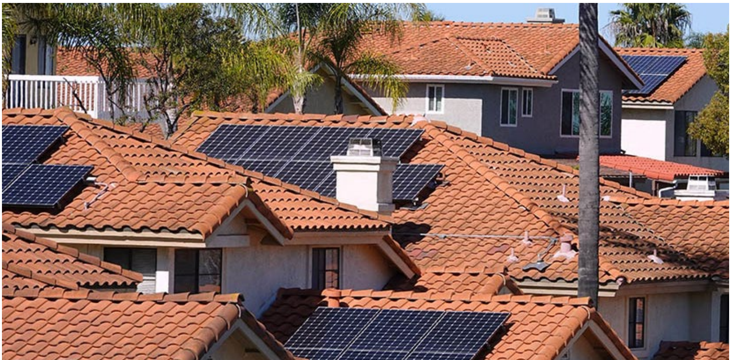
Net metering has incentivized rooftop solar in California. | Shutterstock
