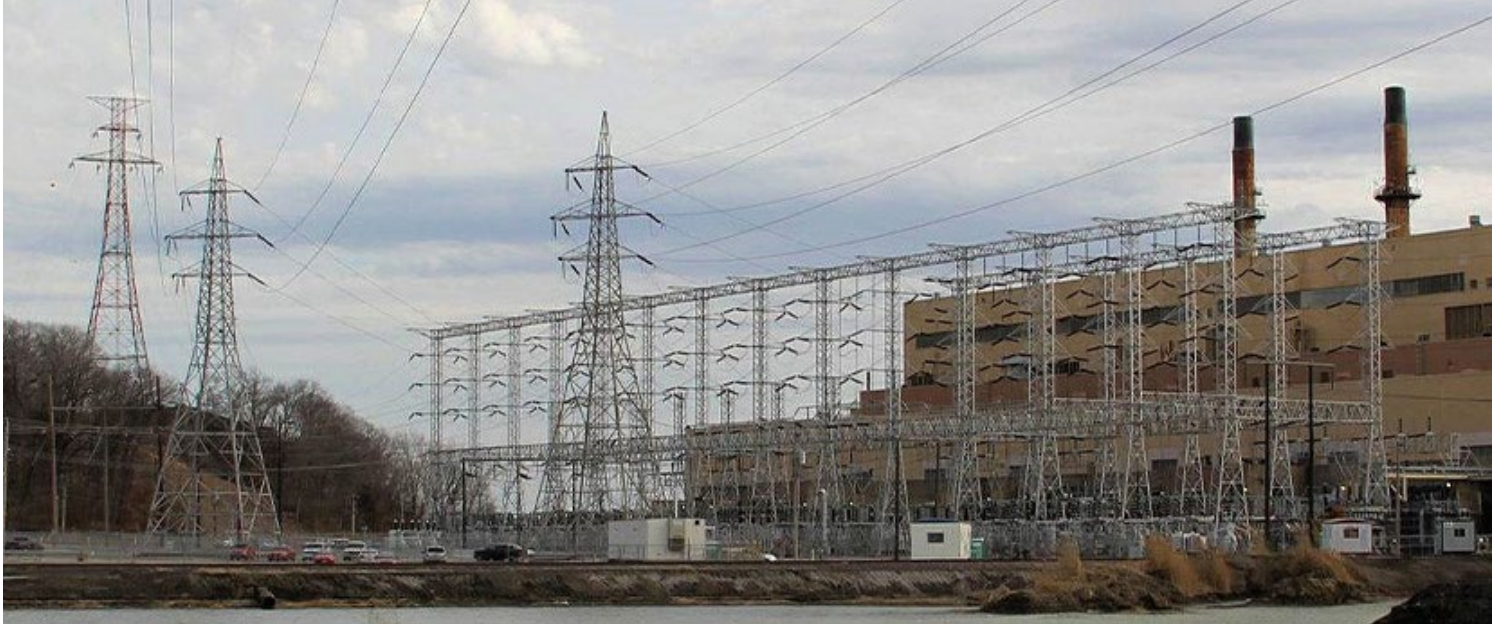
Ameren's coal- and gas-fired Meramec Power Plant | Missouri State Representative Jim Murphy
