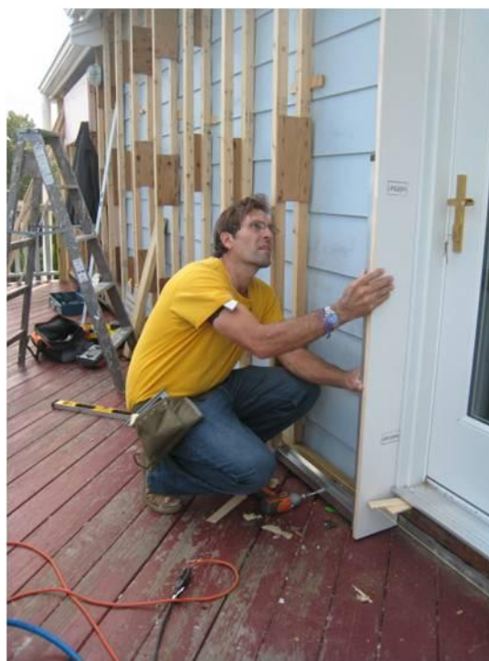
Deep retrofit with super-insulation. (source: DOER)
