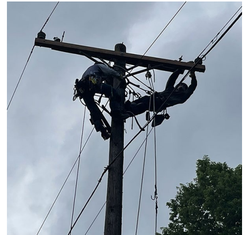
AEP Ohio linemen work to restore power. | AEP Ohio
