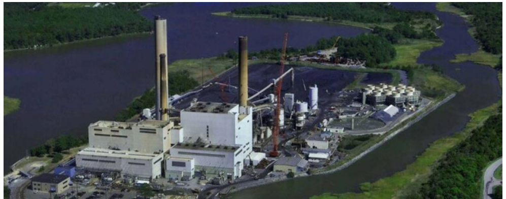
The announcement of the planned closure of NRG’s Indian River Generating Station in Delaware was one of several generating unit deactivation notifications in PJM last summer. | NRG
