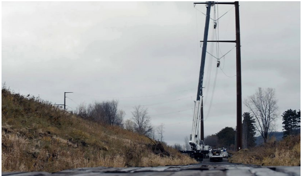
Construction of the MISO MVP Badger-Coulee project in Wisconsin | IBEW
