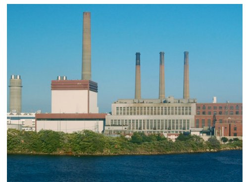
Mystic Generating Station
