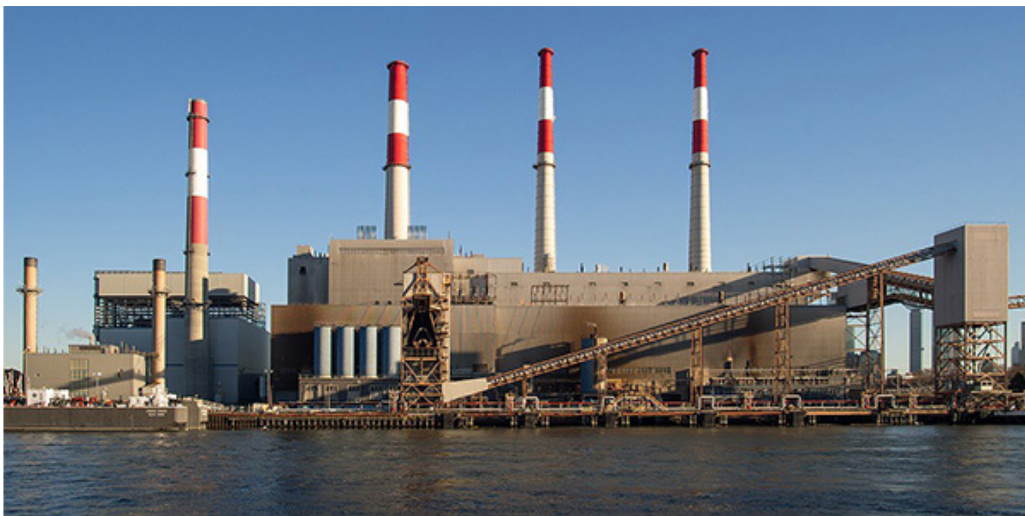
The 2,480-MW Ravenswood Generating Station in Queens, N.Y.
