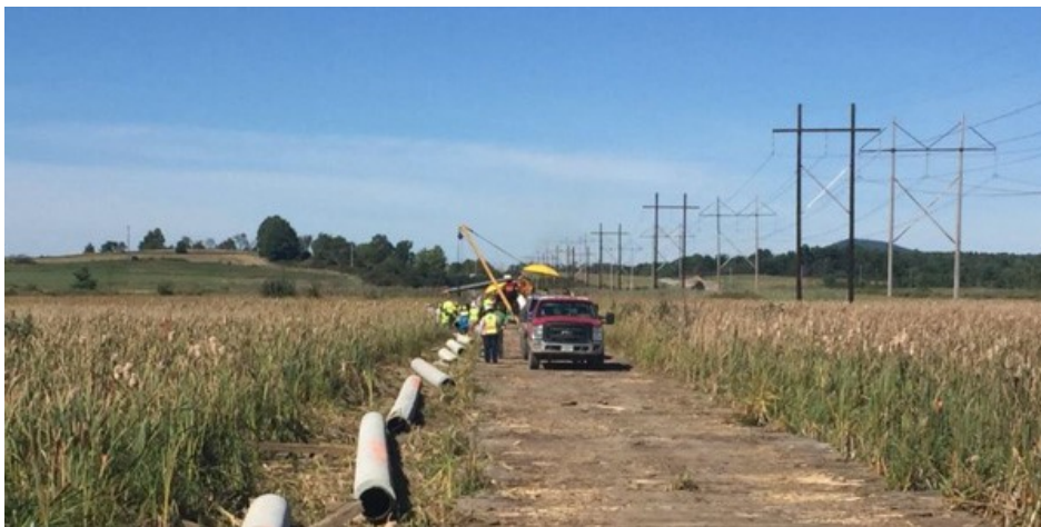
Addison natural gas project construction | VHB
